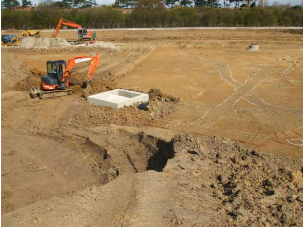
Plate 2. The central south-western part of the site looking north during the site strip
